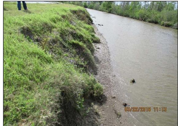
The existing levee elevation ranges from +6.0 feet to +7.5 feet (average elevation of approximately +7.0 feet) with side slopes of 1 vertical to 3 horizontal (1V on 3H) and a crown of varying width. The existing levee was constructed using cohesive soil on the canal side and riprap (stone) was then later installed along the pond side.
