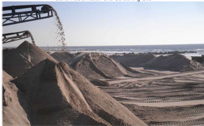
Clean Sand Coming Off the Screen onto the Beach
