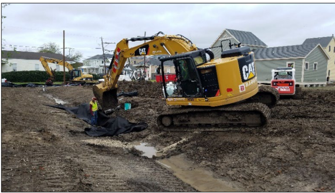
Figure 1: Grading and construction of the bioswale systems
