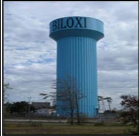
**Elevated Water Storage Tank No. 3; East Biloxi:** Design, bidding, and construction administration for a **one (1) million gallon elevated water storage tank.** N-Y utilized the EPA.Net Program to model the water system for the East Biloxi area to confirm the capacity and elevation of the water tank.
