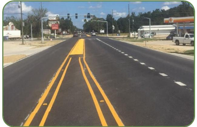
The project consists of *asphaltic concrete pavement widening of 1,800' along LA 431 and 400' along LA 934.*
