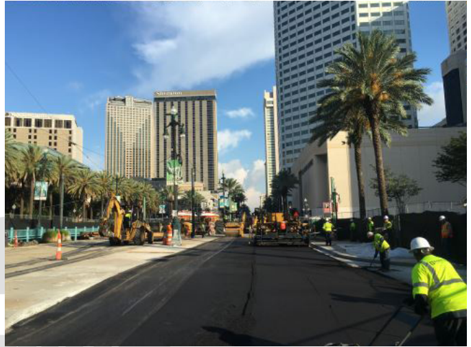
Figure 3. Our team served as the Owner's Representative and provided emergency professional engineering services for the Expressway Tunnel Collapse on Canal Street in New Orleans, LA. Our structural engineers provided a fast pace approach to repairing the damaged tunnel end wall while coordinating with our transportation engineers designing the roadway and street car repairs to reopen the roadway within 46 days of collapse.
