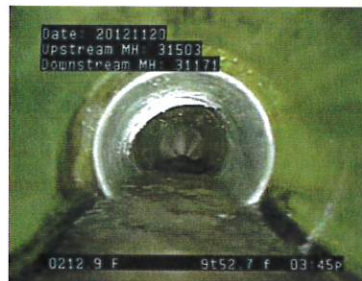
After Lateral Rehabilitation
