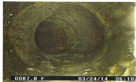
CIPP Lateral after 15 months in Service
