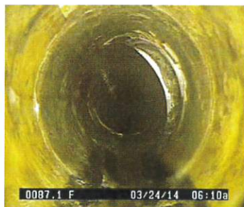
CIPP Lateral after 15 months in Service
