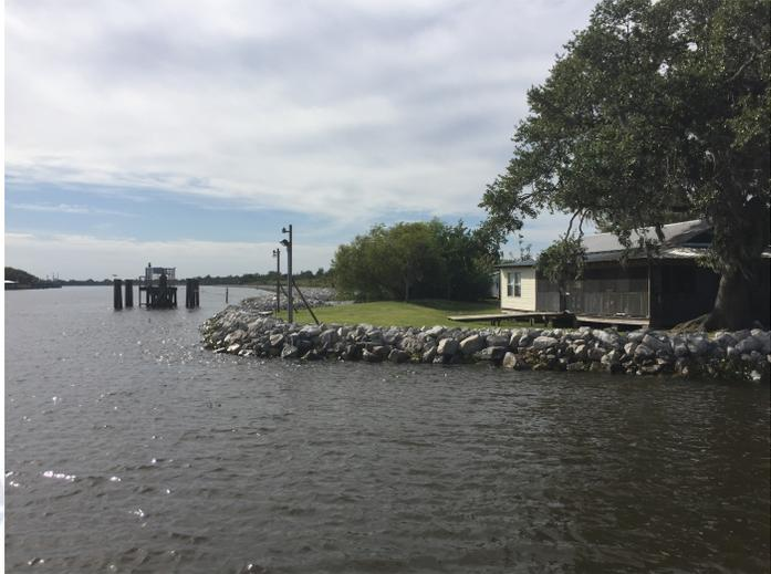
The project consists of approximately 10,600 linear feet of foreshore rock dike to protect the west bank of the Barataria Waterway and adjacent interior marshes from Bayou Rigolettes south to the existing CWPPRA shoreline protection project. Additional shoreline protection was constructed on the north shoreline of Bayou Rigolettes at Bayou Barataria to eliminate shoreline erosion and protect the Grand Isle water storage tank which is located on the peninsula.
