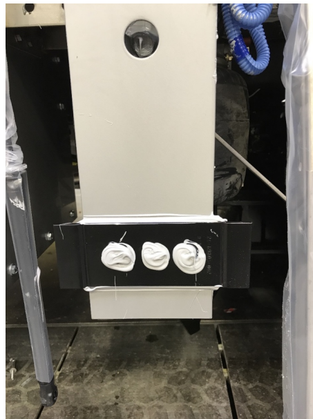
Sealed & powder coated aluminum skirt panel bracket
