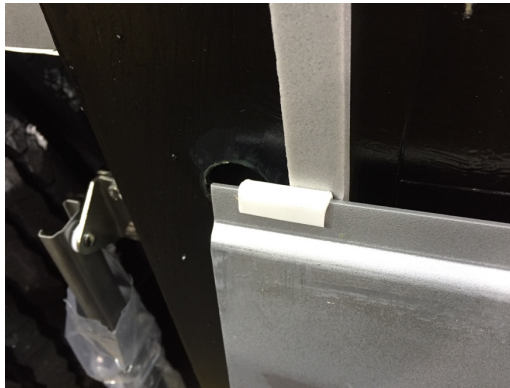
Tape applied to top edge of coated skirt panel
