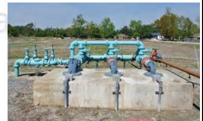
Dalcour WTP Service Pumps and Manifold
