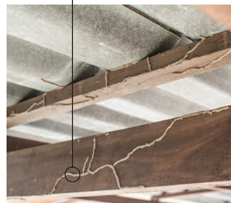
Termite damage to wood
