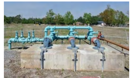
Dalcour WTP Service Pumps and Manifold
