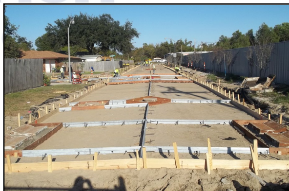
Looking East towards Queens Blvd. ready for concrete replacement
