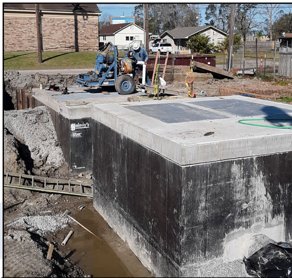
Wet Well & Valve Box for the Pump Station
