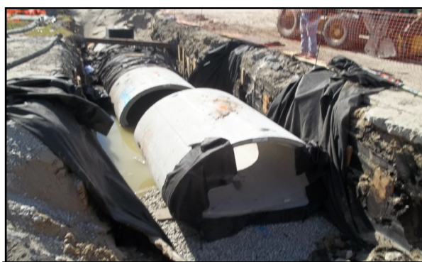
Installed 45"x73" RCPA drainage culvert
