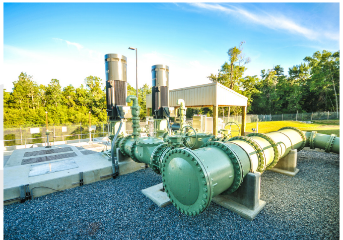
Figures 1 and 2. Our team designed a new raw water intake and pumping facility to provide increased redundancy and reliability to the current Bay County, FL water supply system. The new facilities for the Alternate Water Supply included the following major equipment and structures: 30 MGD triplex vertical turbine pump station (1,800 hp total); 10 miles of 36-inch raw water main; and passive intake facility with screens, back-up generator power, and telemetry.
