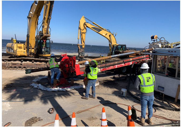
Figure 4. When Bay County, FL was undertaking their largest trenchless project to-date and needed a trusted advisor, they selected Mott MacDonald as Owner's Representative and Resident Engineer to oversee the design and construction for this 5,290-foot-long 24-inch HDD underneath St. Andrews Bay.
