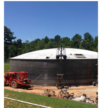
Figure 8. Water storage facility for the Central Elmore Water and Sewer Authority, which included two new 1 MGD pre-stressed concrete clearwell ground storage tanks, 24-inch DI pipe, electrical, and SCADA systems, associated site work, and demolition of existing facilities.
